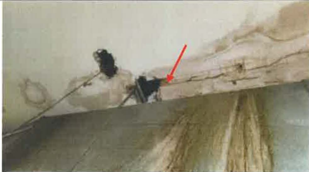
Sample location for asbestos drywall compound (A-3 & 4)
