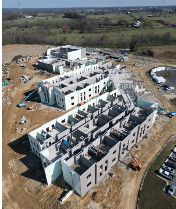
Aerial View of Building
