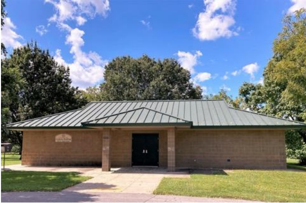
Coolavin Park 550 W. 6 th St. • 40508 1 st District
